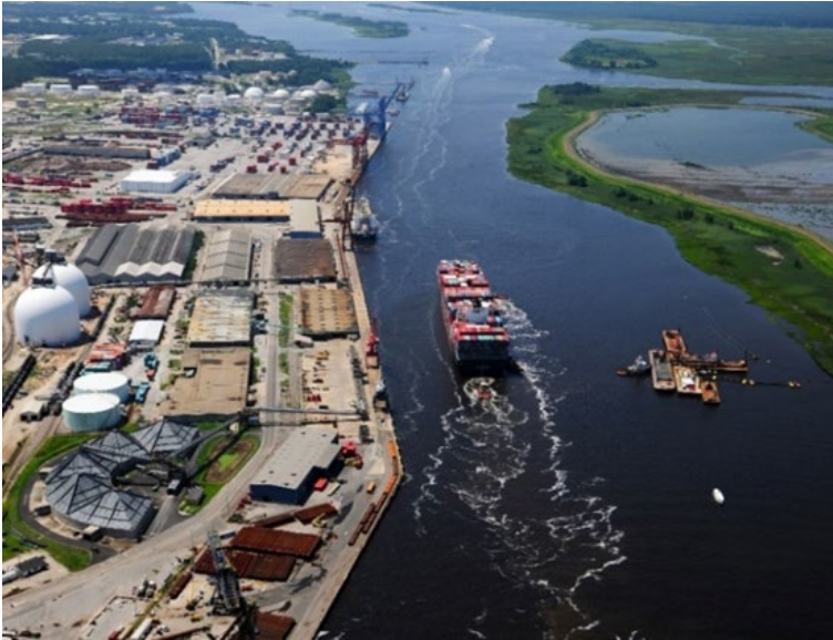
FIGURE 2.2 AERIAL PHOTO OF PORT OF WILMINGTON
