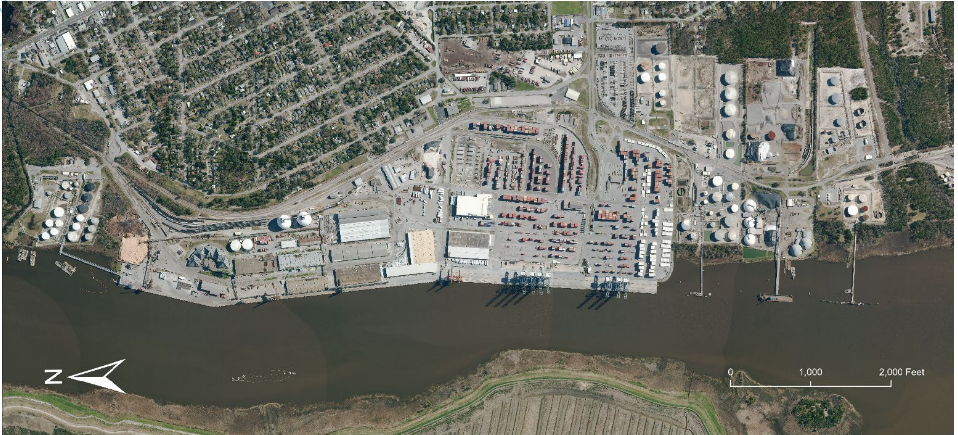
Port of Wilmington Aerial
